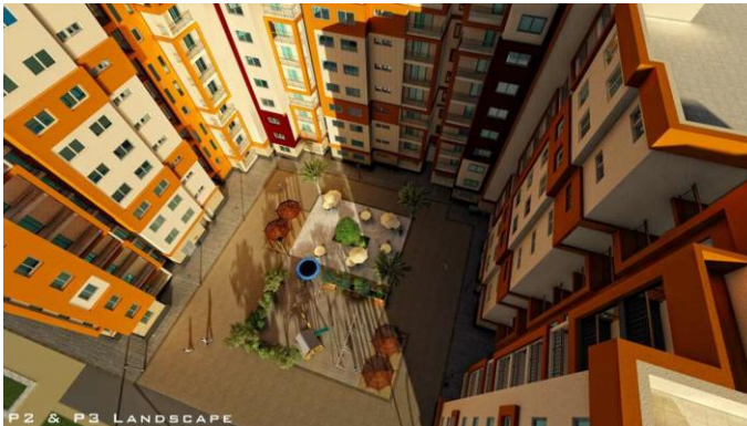
PUBLIC HOUSING | SHARED COURTYARD VIEW
